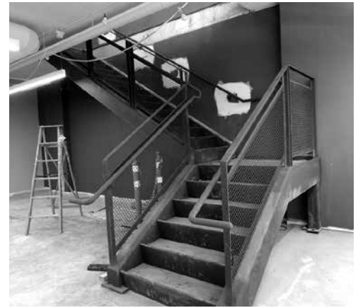
View of stairs from ground floor.
