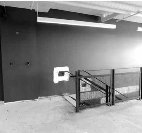
View of stairs from upper floor.
